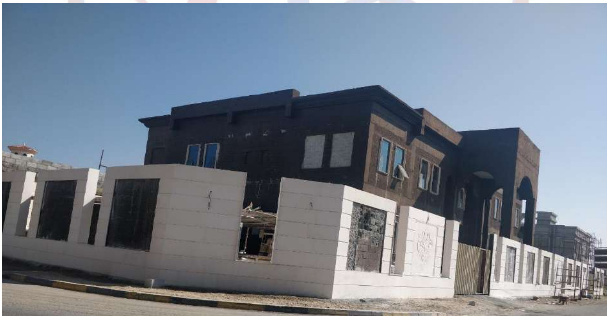
Mr. Seed (G+1) Villa at Fujairah, ARCOTIS Brand , M.R.L Passenger Elevator, Speed: 1.0 (m/s), Capacity: 630 KG/8persons.
