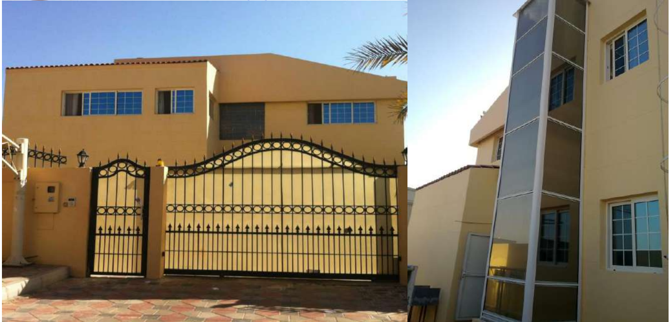
Mr. Abdulla Sultan Al Sharhan (G+1) Villa at Merdif – Dubai, ARCOtis Brand, Hydraulic Home Elevator, Speed: 0.4 (m/s), Capacity: 260 KG/3persons.
