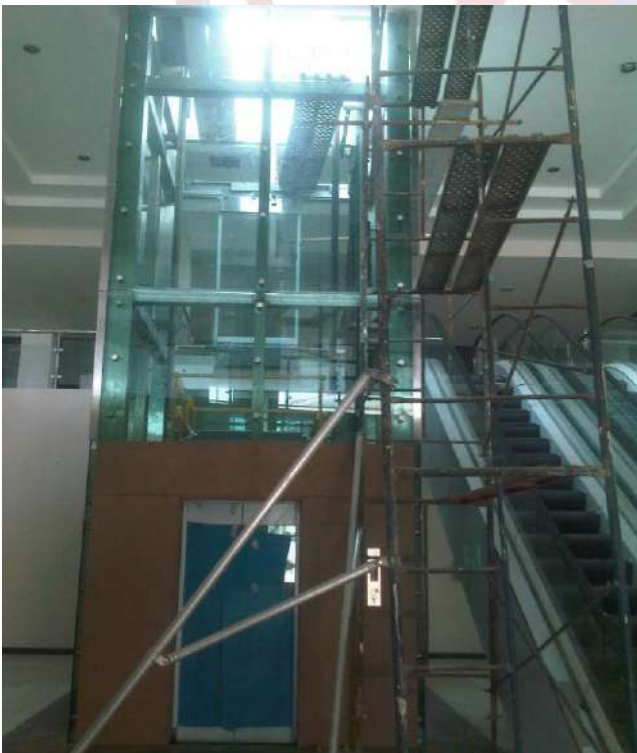
M/s. Dubai Investment Park (G+1) Community Center at D.I.P, ARCOTIS Fuji Brand , 2Nos. Escalators & M.R.L Panoramic Passenger Elevator, Speed : 1.0 (m/s), Capacity: 800 KG/10persons.
