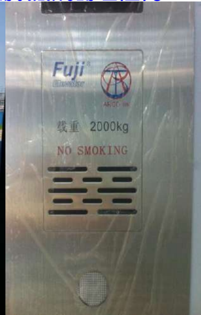
M/s. Al Hoot Contracting Throw M/s. Safeline Gent. Maint. Cont., (G+1) at Dubai Crown Prince Farm -Al Barsha-Dubai, ARCOTIS Fuji Brand , Hydraulic Forklift Elevator, Speed: 0.6 (m/s), Capacity: 2000 KG.
