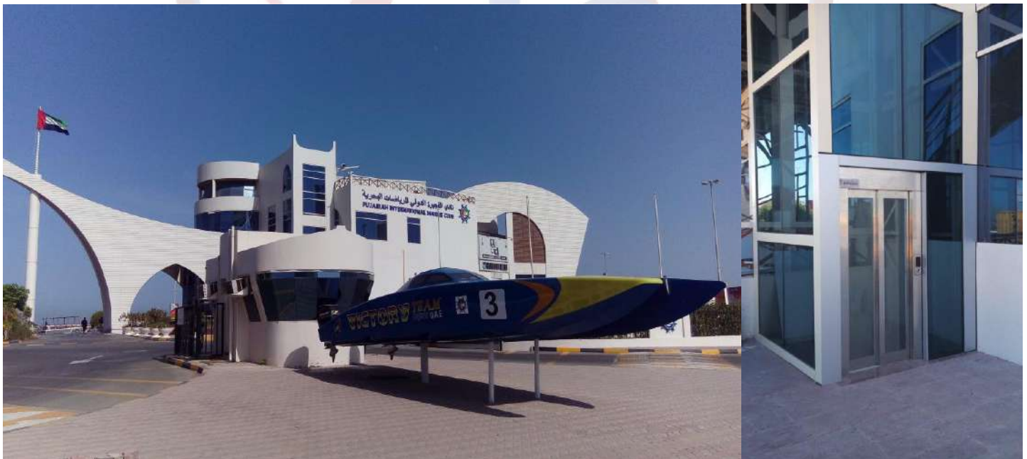
M/s. Fujairah International Marine Club / M/s. RJJ's Restaurant Fujairah (G+2) Building at Fujairah, ARCOtis Brand, Hydraulic Panoramic Passenger Elevator, Speed: 0.6 (m/s), Capacity: 450 KG/6persons.
