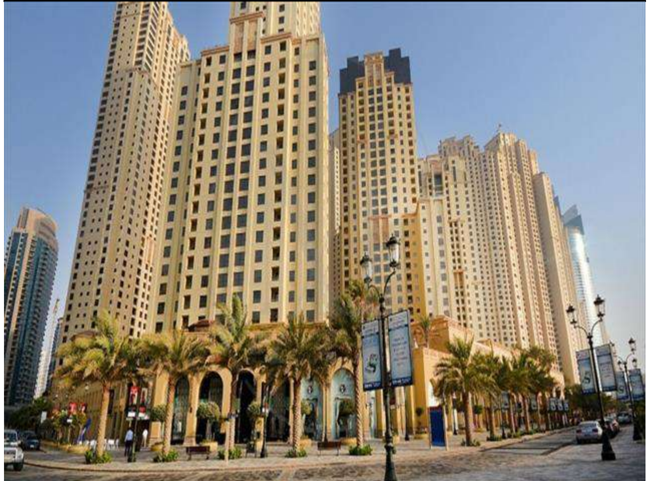
M/s. HAWTHORN Suites By Wyndham (G+1) at J.B.R-Dubai, ARCOTIS Brand, Dumbwaiter Lift, Speed: 0.35 (m/s), Capacity: 150 KG.
