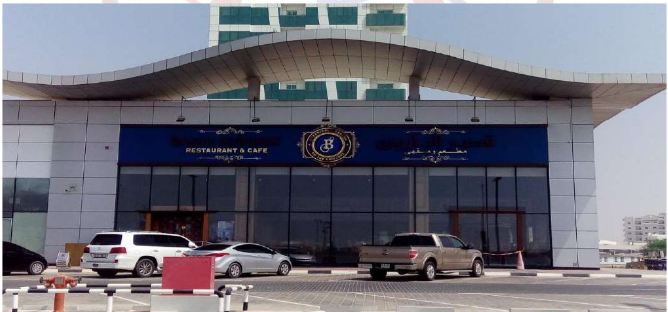
M/s. QASAR AL BARON Restaurant & Cafe (G+1) at Ajman, ARCOTIS Brand , Dumbwaiter Lift, Speed: 0.30 (m/s), Capacity: 100 KG.
