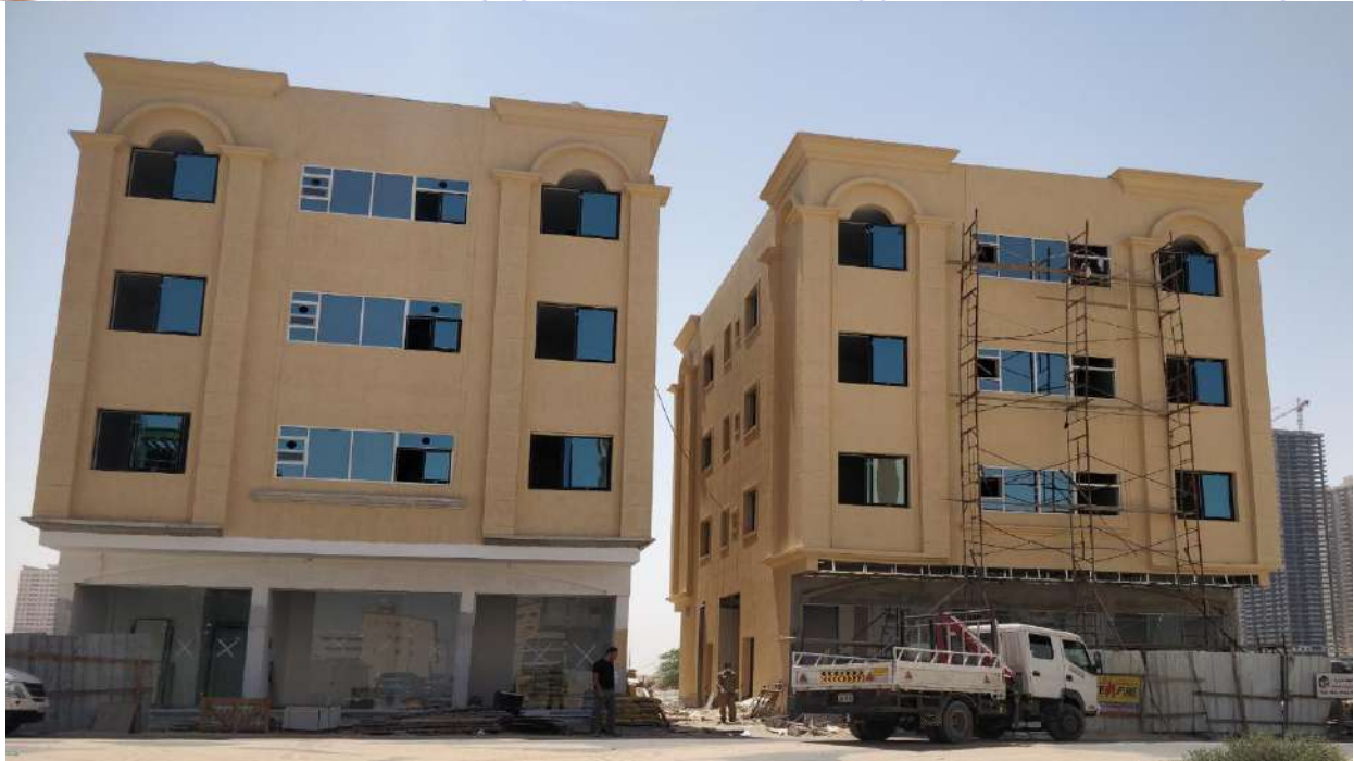
M/s. Al Rasikhoon Real Estate / M/s. Rihlat Alomr Building Contracting, Two (G+3) Buildings at Alia - Ajman, ARCOTIS Fuji Brand , M.R Passenger Elevators, Speed : 1.0 (m/s), Capacity: 630 KG/8persons.
