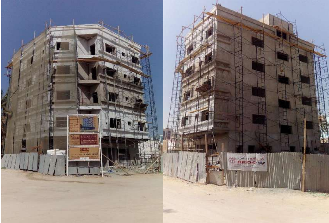
M/s. Al Turath Al Omrani Engineering Consultants / M/s. Afaq Al Sharq Building Contracting (G+4) Building at Ajman, ARCOTIS Fuji Brand , M.R Passenger Elevator, Speed : 1.0 (m/s), Capacity: 450 KG/6persons.
