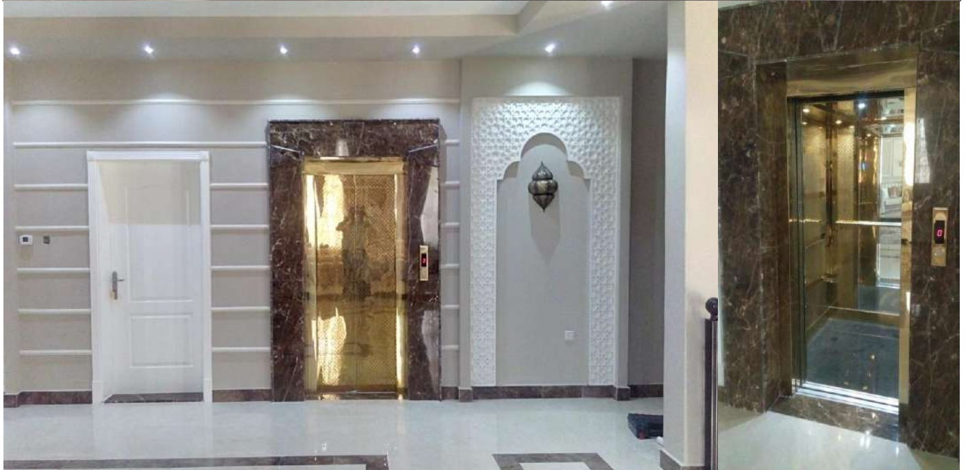
M/s. Al Turath Al Omrani Engineering Consultants / M/s. Afaq Al Sharq Building Contracting (G+1) Villa at Ajman, ARCOtis Brand , Hydraulic Golden Passenger Elevator, Speed: 0.6 (m/s), Capacity: 630 KG/8persons.
