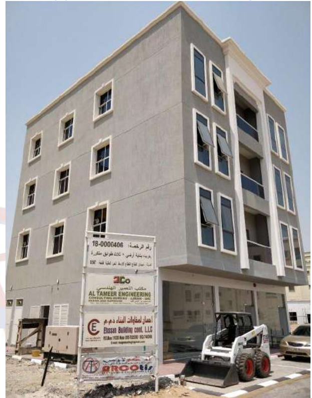
M/s. Al Tameer Engineering Consulting / M/s. Ehssan Building Cont. (G+3) Building at Ajman, ARCotis Brand , MR Passenger Elevator, Speed: 1.0 (m/s), Capacity: 630 KG/8persons.
