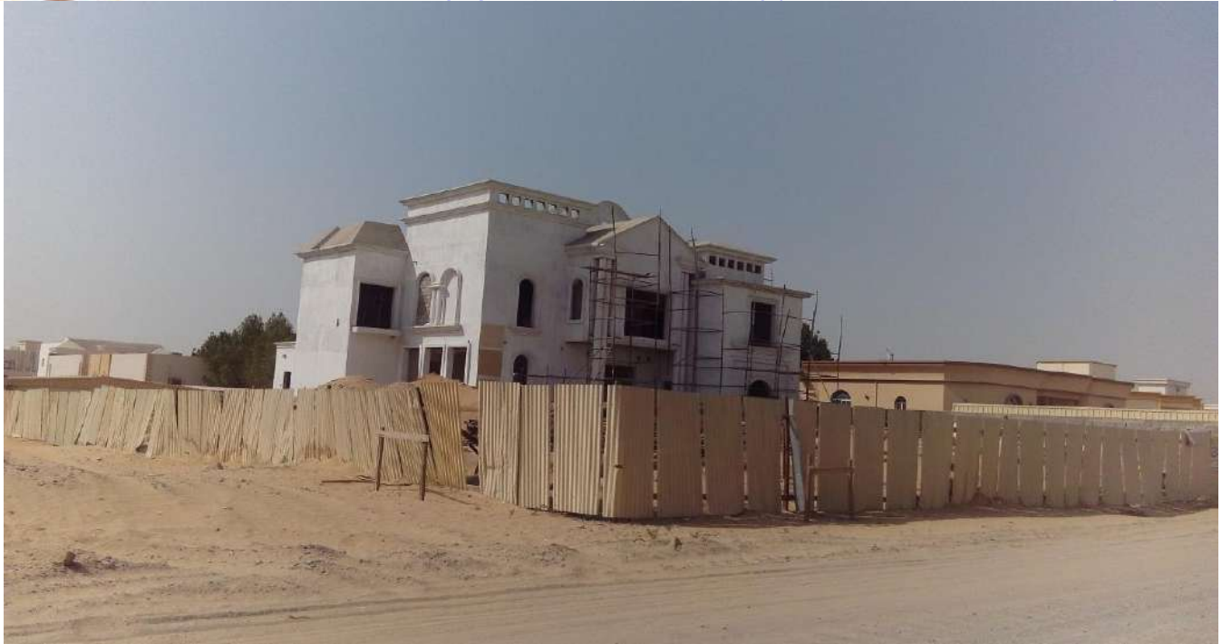
M/s. Deyar Engineering & Consultants / Mr. Omar Al Durs (G+1) Villa at Al Nouf 2-Sharjah, ARCOtis Brand, Hydraulic Passenger Elevator, Speed: 0.6 (m/s), Capacity: 450 KG/6persons.
