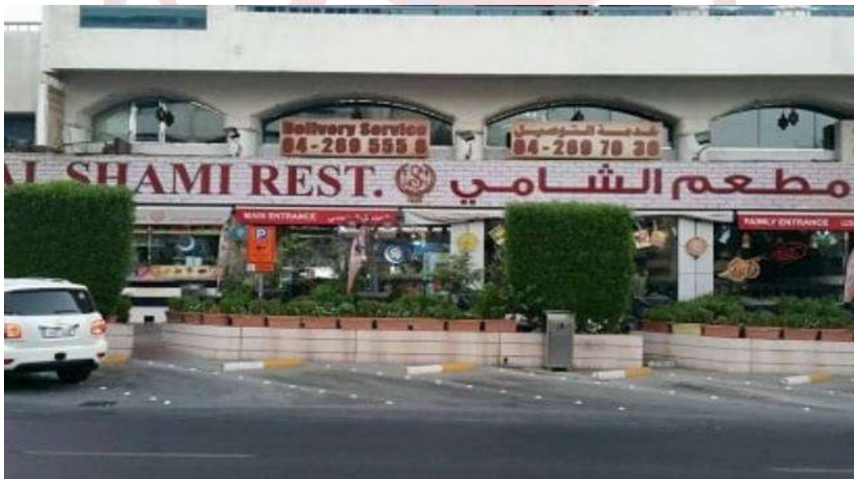
M/s. Al Shami Restaurant (G+1) Restaurant at Al Murakabat– Dubai, ARCOTIS Brand, Dumbwaiter Lift, Speed: 0.3 (m/s), Capacity: 200 KG.
