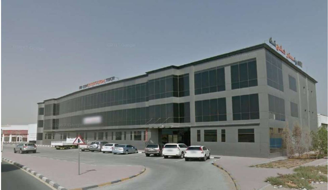
M/s. Rehlat Al Omr Building Contracting (G+2) Offices Building at Ajman, ARCOtis Fuji Brand, Golden MRL Semi Round Home Elevator, Speed: 1.0 (m/s), Capacity: 630 KG/8persons.
