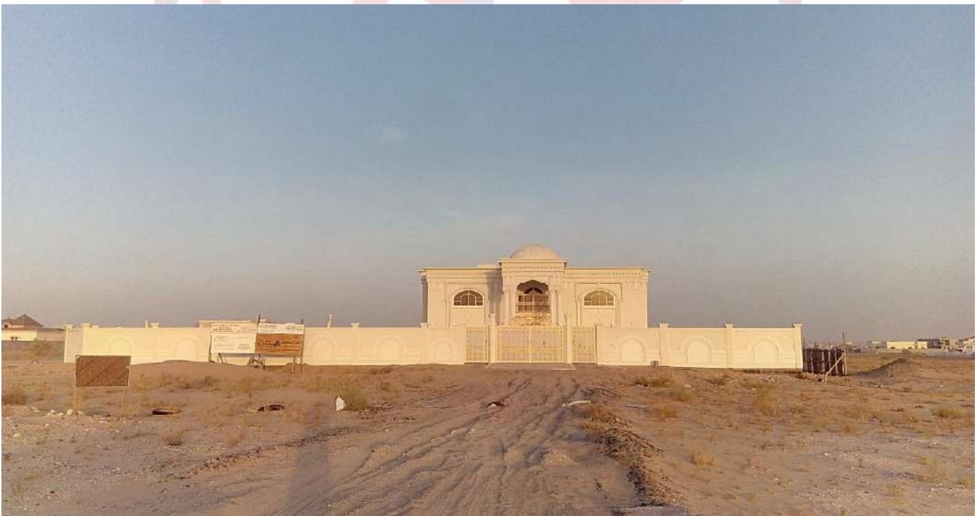
M/s. Concord Engineering Consultants / M/s. Al Fan Al Muasir Building Cont. Co. LLC (G+1) Villa at Al Seyoh- Sharjah, ARCOtis Brand, M.R Golden Passenger Elevator, Speed: 1.0 (m/s), Capacity: 450 KG/6persons.
