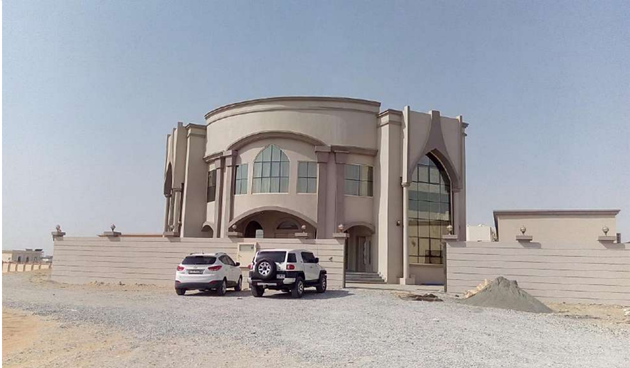
M/s. Alhilal Engineering Consultants /M/s. Ruayat Building Contracting /Mrs.Mariam Al Hammdi (G+1) Villa at Rahmaniya-Sharjah, ARCOTIS Brand , Hydraulic Passenger Elevator, Speed: 0.6 (m/s), Capacity: 320 KG/4persons.
