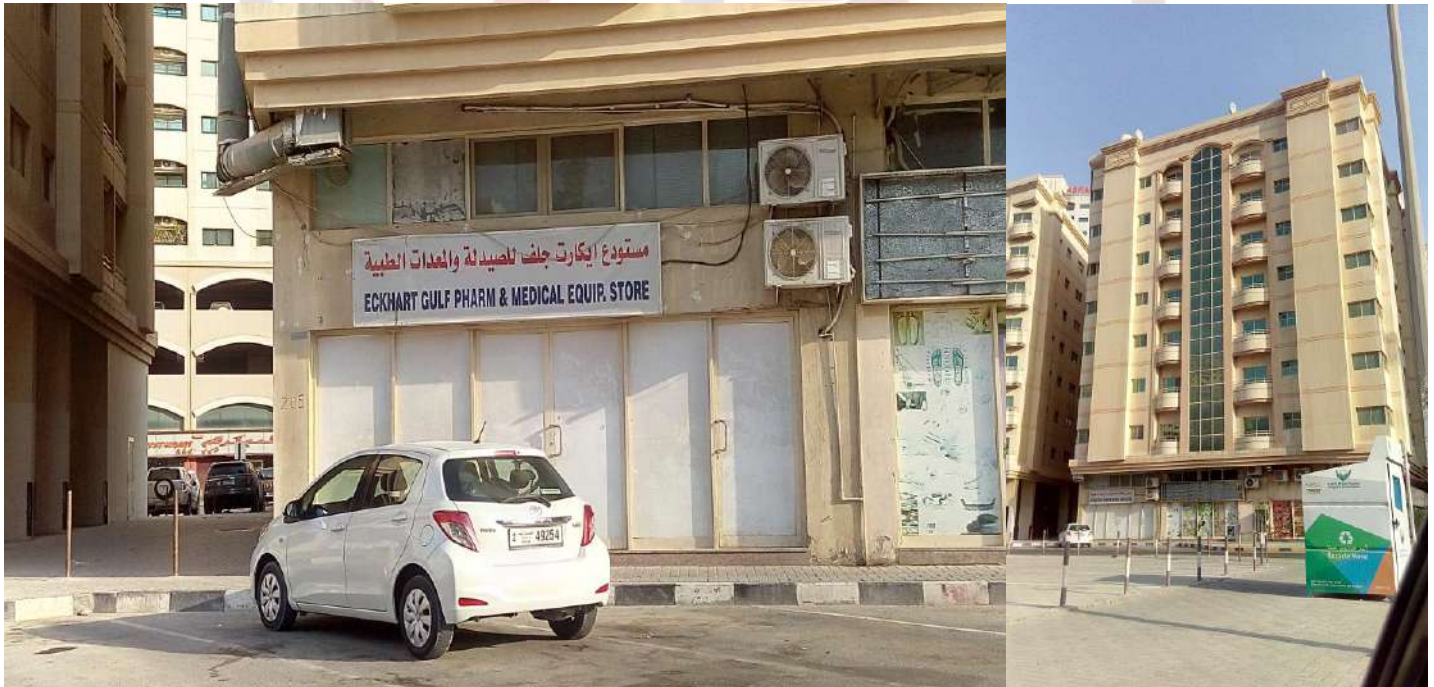
Dr. Ahmad (G+M) Warehouse at Sharjah, ARCOtis Brand, Platform Lift, Speed: 0.35 (m/s), Capacity: 600 KG.
