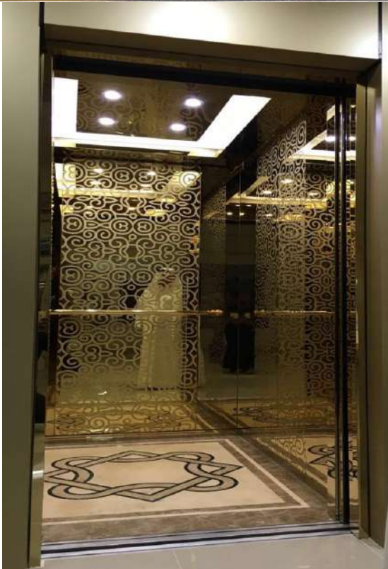
Mr. Saeed Al Shamsi (G+1) Villa at Al Rahmanyah 7 – Sharjah, ARCOtis Fuji Brand, M.R.L Passenger Elevator, Speed: 1.0 (m/s), Capacity: 450 KG/6persons.
