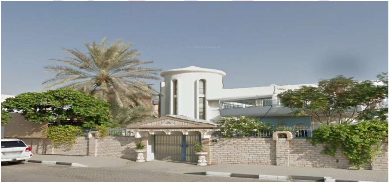
Mr. Khalid Al Amoudi, (G+1) Villa at Sharjah, Two Lifts (ARCOtis Brand, Hydraulic Elevator, 3 Phase, Speed: 0.6 (m/s), Capacity: 450 KG/6persons) & (ARCOtis Fuji Brand, Semi Round Hydraulic Home Elevator, Speed: 0.3 (m/s), Single Phase, Capacity: 400 KG/4persons).
