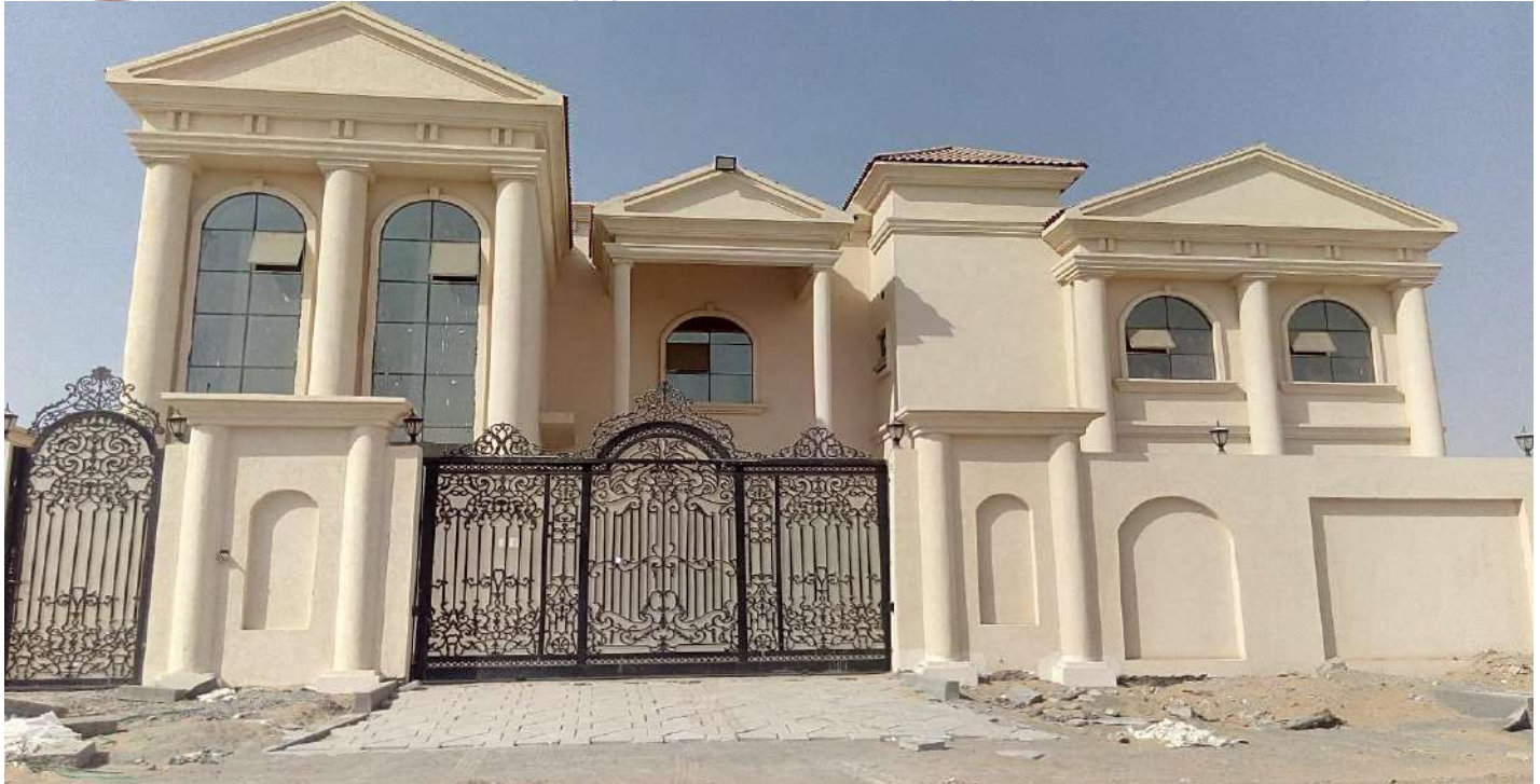
M/s. Deyar Engineering & Consultants / Dr. Adil Abdullah Khamis Al Maimari (G+1) Villa at Rahmaniya-Sharjah, ARCOtis Brand , Hydraulic Passenger Elevator, Speed: 0.6 (m/s), Capacity: 630 KG/8persons.
