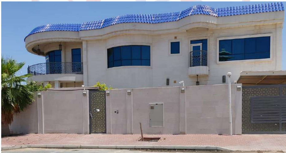
Al Salam Building Contracting / Mr. Naji (G+1) Villa at Tawar – Dubai, ARCOtis Brand, Hydraulic Home Elevator, Speed: 0.3 (m/s), Single Phase, Capacity: 2600 KG.
