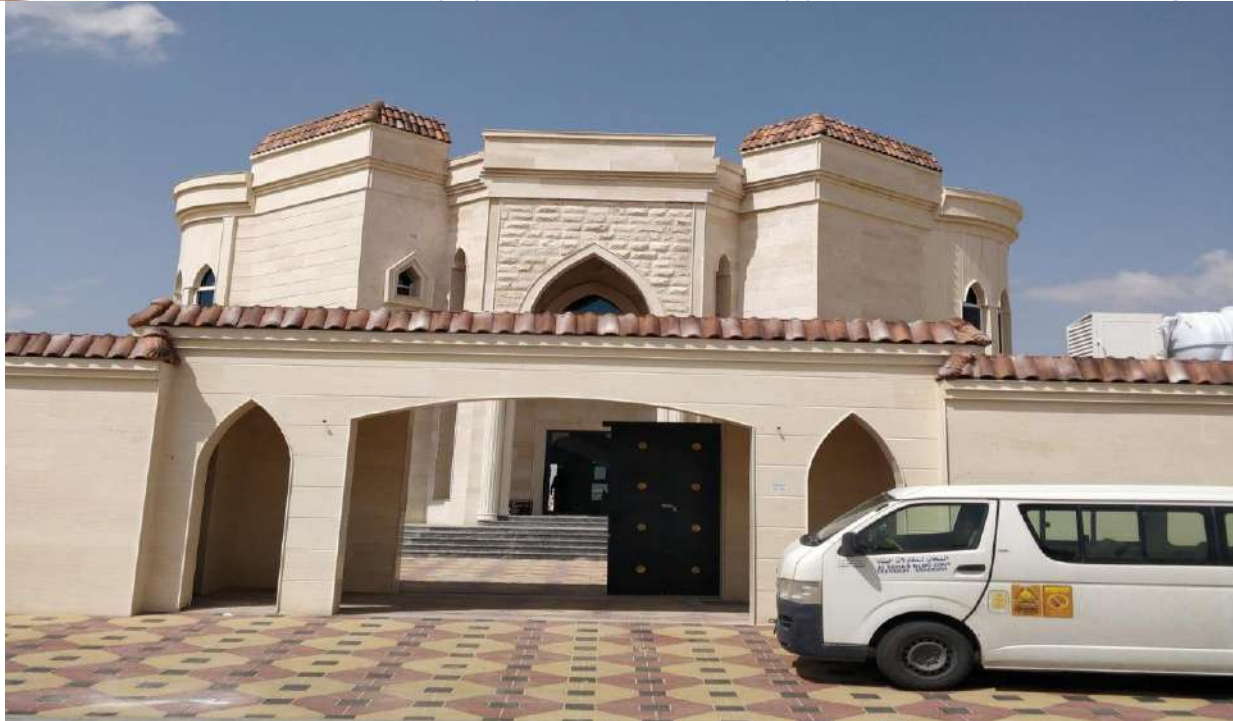
M/s. Al Ruayah Al Thakiah Eng. Consultants L.L.C / Mrs. Zahra Al Alawi (G+1) Villa at Sharjah, ARCOtis Brand, Hydraulic Passenger Elevator, Speed: 0.6 (m/s), Capacity: 450 KG/6persons.
