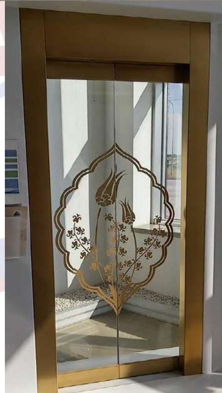
Mr. Saeed Al Shamsi (G+1) Villa at Al Rahmanyah 7 – Sharjah, ARCOtis Fuji Brand, M.R.L Passenger Elevator, Speed: 1.0 (m/s), Capacity: 450 KG/6persons.
