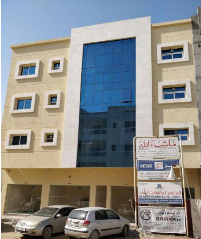
M/s. Deyar Engineering & Consultants / M/s. AlMughamir Bldg. Cont. (G+3) Building at Sharjah, ARCOTIS Brand , MR Passenger Elevator, Speed: 1.0 (m/s), Capacity: 630 KG/8persons.
