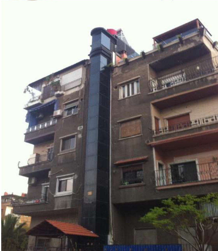
(G+3) Building, MR Panoramic Passenger Elevator, At Damascus-Syria , ARCOTIS Brand
