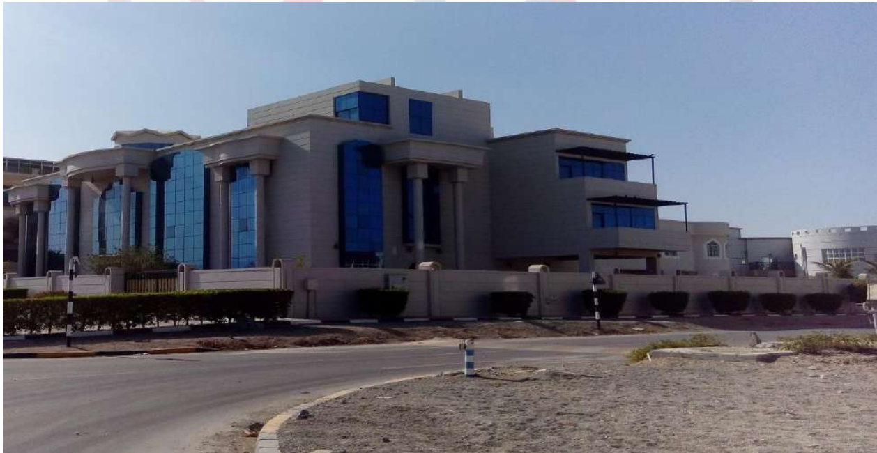
Mr. Fahad Salem Al Hosani (G+1) Villa at Abu Dhabi, ARCOTIS Brand , Hydraulic Home Elevator, Speed: 0.4 (m/s), Capacity: 450 KG/6persons.
